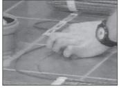
the mesh and loops formed manually, but ensure the cables are spaced the same distance as those on the mat.
