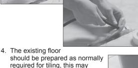
required for tiling, this may include cleaning and removing all loose particles. removing any sharp protrusions that may cause damage to the heating wire. priming the floor surface and bracing a timber floor with WBP
